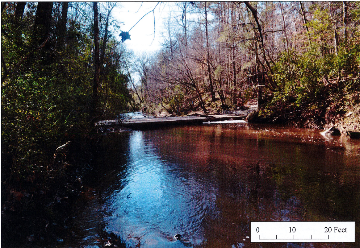
Photograph 3. Looking South Downstream to Densons Creek Vented Ford
