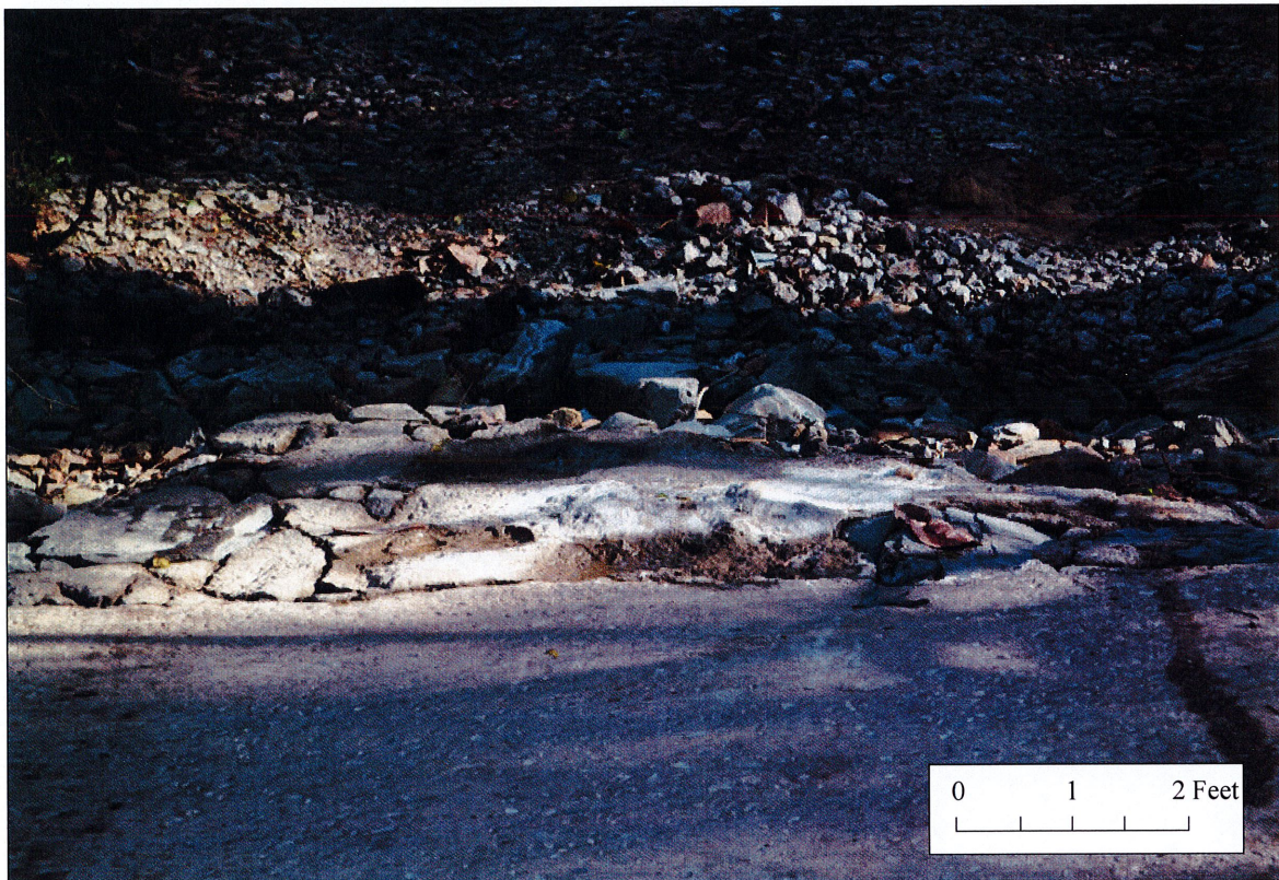
Photograph 10. Fill at East Embankment
