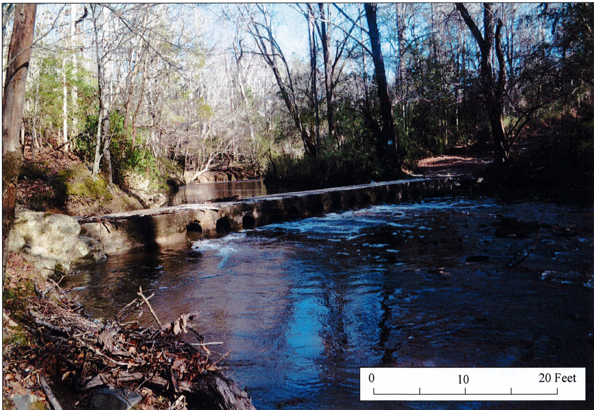
Photograph 4. Looking North Upstream to Densons Creek Vented Ford
