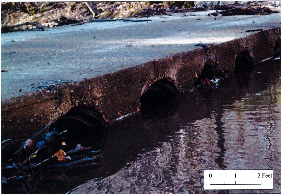
Photographs 9. Detail of Culverts
